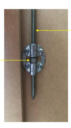
Tension Rod on back of sliding door
